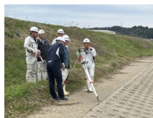
ICT 測量研修
